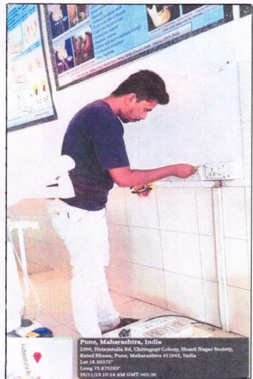
Electrical equipment repair
